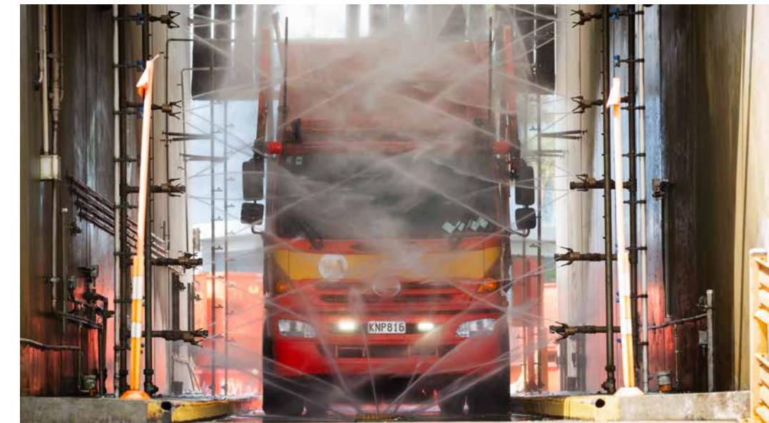
Truck washing using harvested rain water
